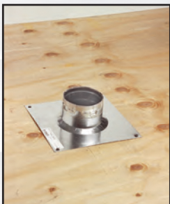
Push pipe through vent support.
