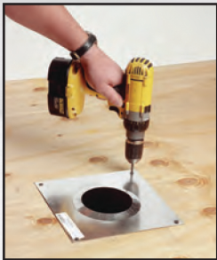
Mount SureGrip support plate.
